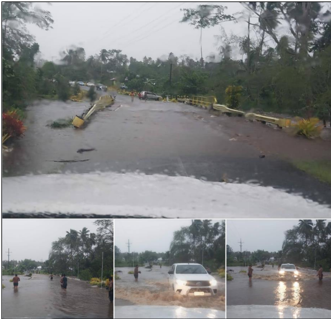
Flooding at Malaemalu, photograph by Land Transport Authority Samoa, 9 March 2025
